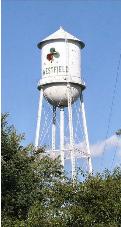
Figure 11: A water tower provides a fluid reservoir at a pressure for the town's water system.
